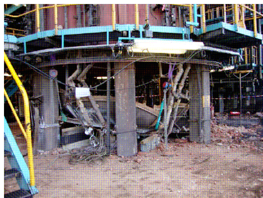
Figure 4 : View of damage sustained on the upper part of the superheater and collapse of the floor plate (DREAL Lorraine)
