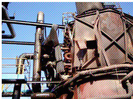
Figure 4 : View of damage sustained on the upper part of the superheater and collapse of the floor plate (DREAL Lorraine)
