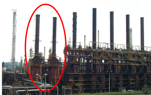
Fig. 2: View of the unit's two superheaters (RR)
